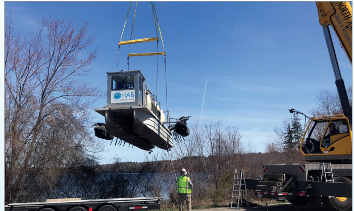
Lowering HAB's Application Barge into Moswansicut Reservoir
